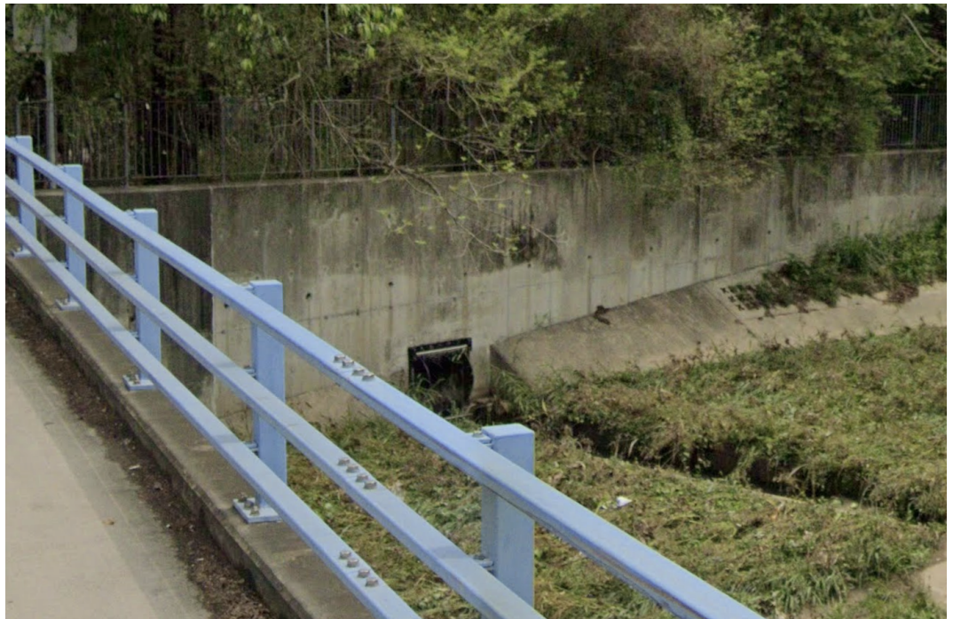
VIEW3: Existing 900mm dia. underground pipe
