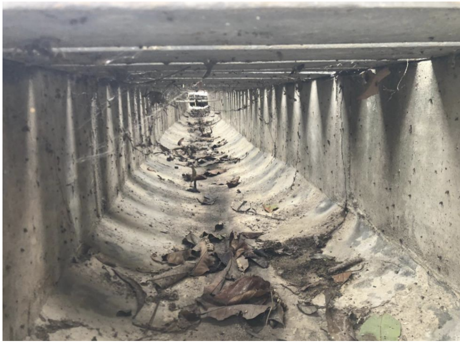
VIEW2: Existing 800UC (Connection)
